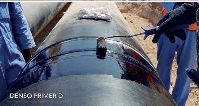
DENSOPOL TAPE PROTECTS THE FIELD JOINTS ON AN OUTFALL PIPELINE
