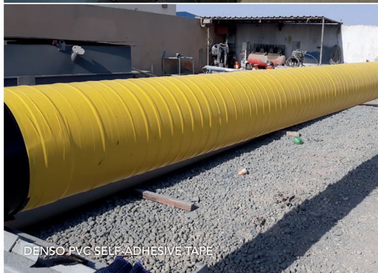
DENSO PVC SELF-ADHESIVE TAPE SPIRALLY WRAPPED OVER DENSOPOL TAPE
