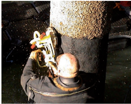
Cleaning with a power tool
