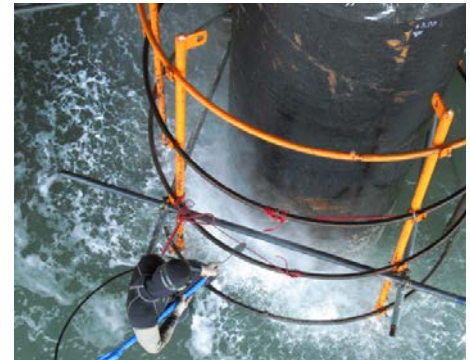
Cleaning using a high pressure water jet
