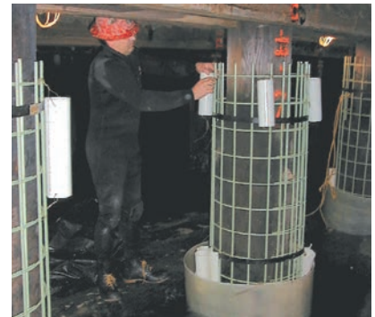
Placing the standoffs around the steel rebars before fitting the Fiber-Forms
