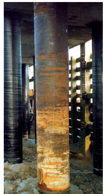
Cleaned pile ready for the application of the SeaShield 80 System
