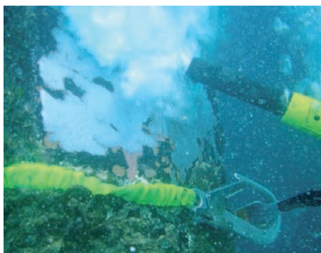
High pressure water jet under water
