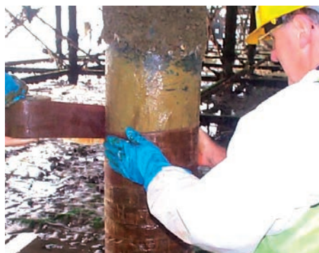
Applying SeaShield Marine Piling Tape
