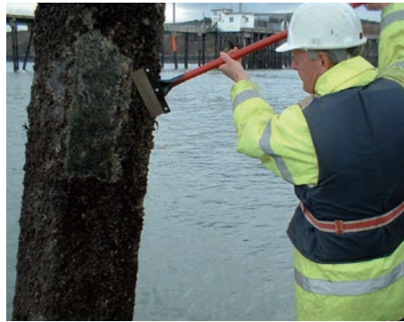
Cleaning with a hand scraper
