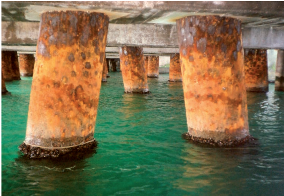
Cleaned piles ready for the application of the Petrolatum Inner Layer
