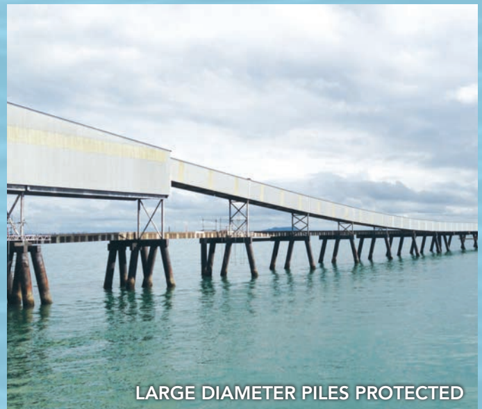
Above: Sugar Loading Jetty, Australia - SeaShield 2000FD System
