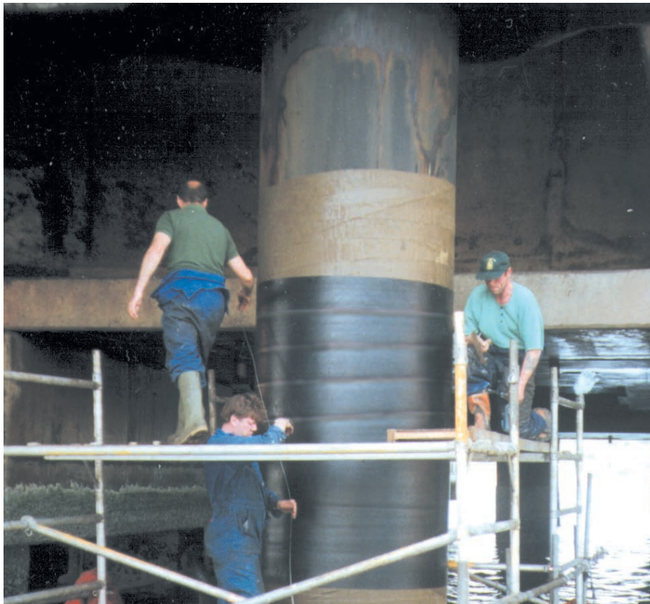
Installing the SeaShield 100 Jackets over the Petrolatum Inner Layer
