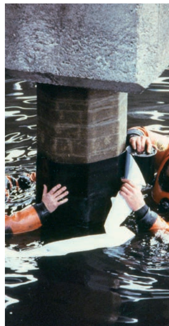
Application of Bitumen Outerwrap Tape 80 over the inner petrolatum tape layer
