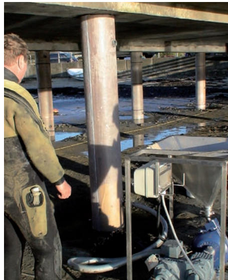
The Epoxy Grout only requires basic pumping equipment
