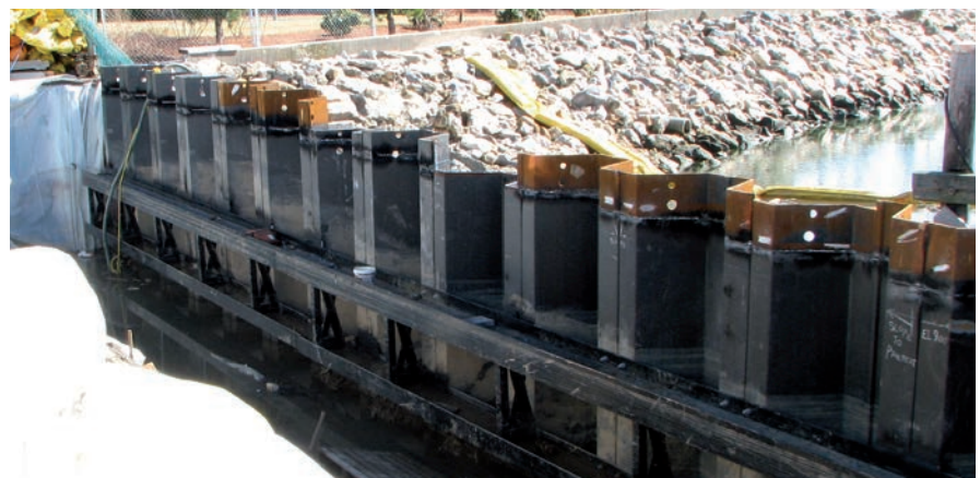
Sheet piling is coated with SeaShield Rigspray prior to being driven into the ground
