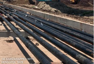
Several corrosion prevention systems are available depending on the condition of the tie bar surface and/or the level of mechanical protection required.
