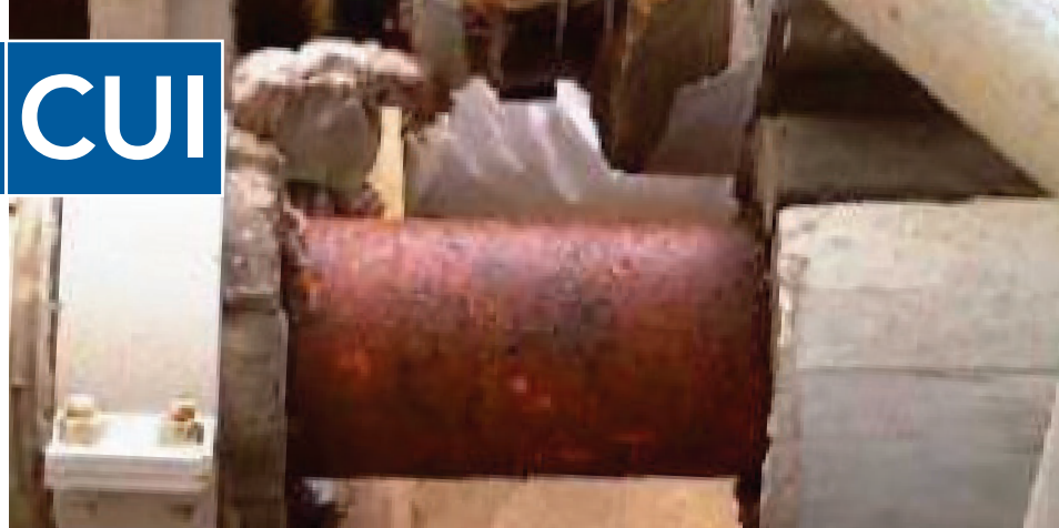
Typical hidden corrosion damage which is often only revealed by removing the pipe insulation!
