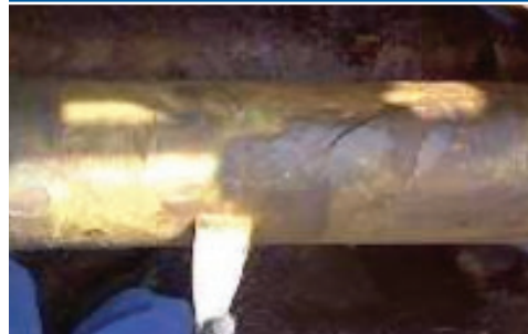
Steelcoat CUI Control System 2: First a layer of Denso Paste...
