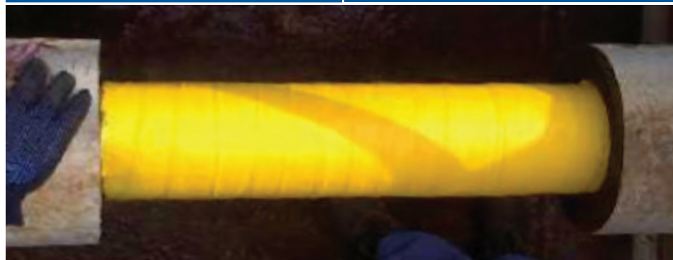
...which is followed by a final layer of Denso PVC Self-Adhesive Tape.
