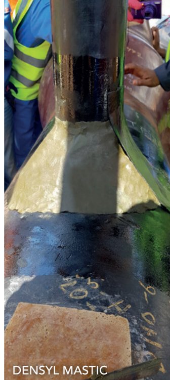
DENSOCLAD TAPE WRAPPED OVER A FLANGE
